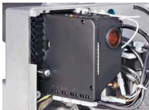
Control box fitted with ignition transformer
