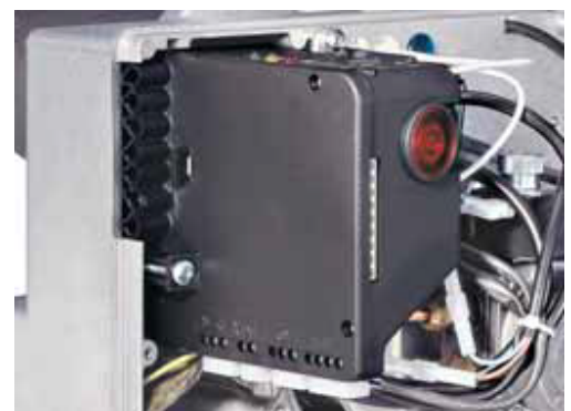
Control box fitted with ignition transformer
